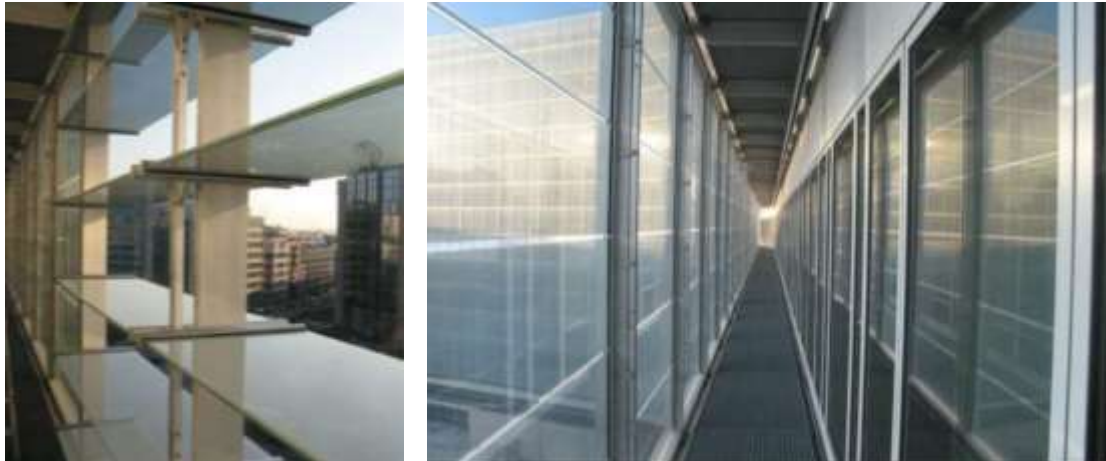
Figure 51 Multi-Story Lower type of Double-Skin Façades. (Lancouer 2004)
