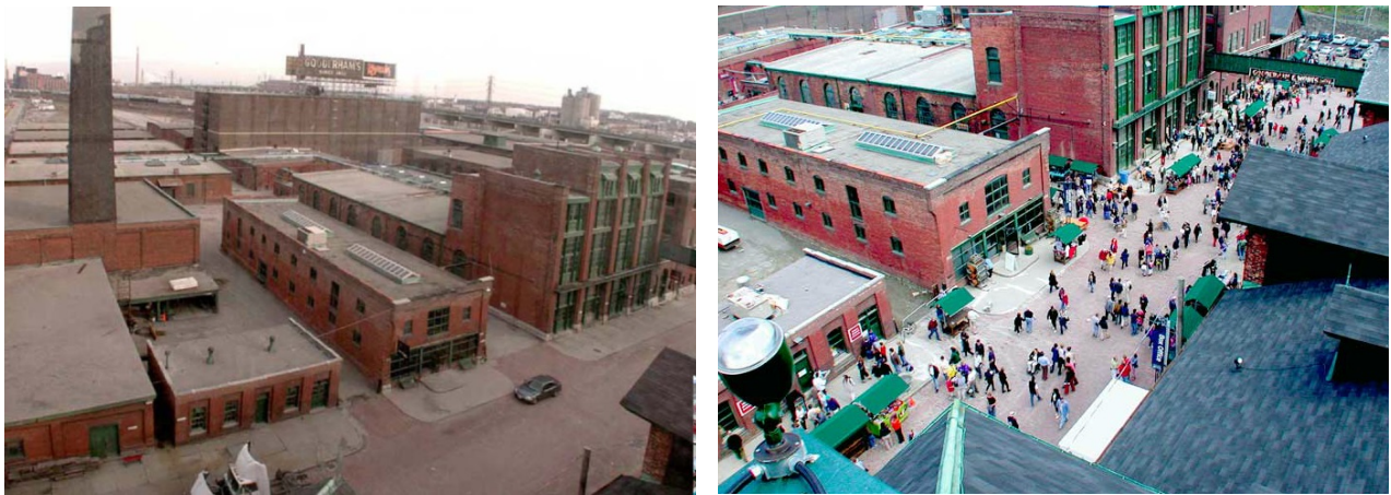
Figure 8 - Distillery District before (right) and after (left) the intervention (source: www.distilleryheritage.com )
