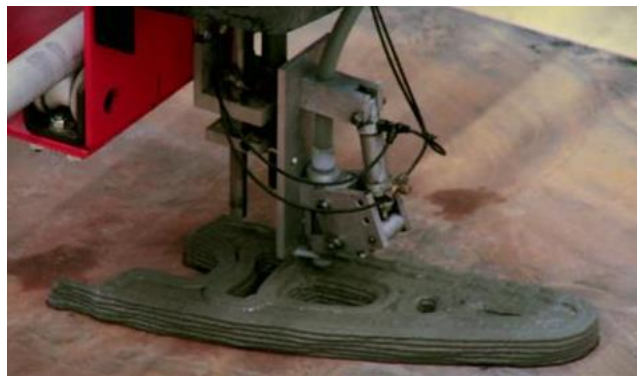
[fig.94] Freeform Construction Project. Loughborough, Reino Unido. Universidad de Loughborough, 2010.
