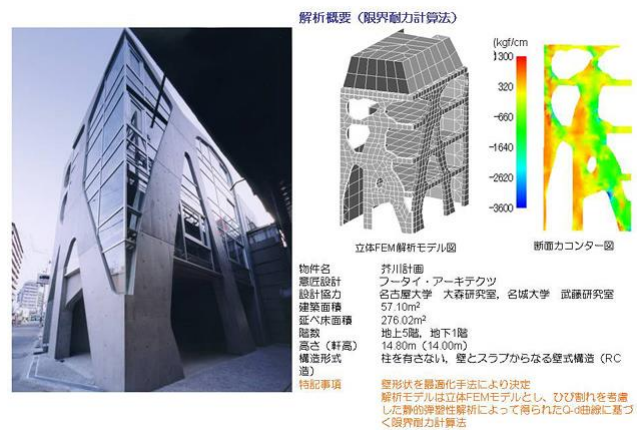
[fig.54] Akutagawa West Side Project. Osaka, Japan. Iijima Architects; Universidad de Nagoia, 2002-2005.
