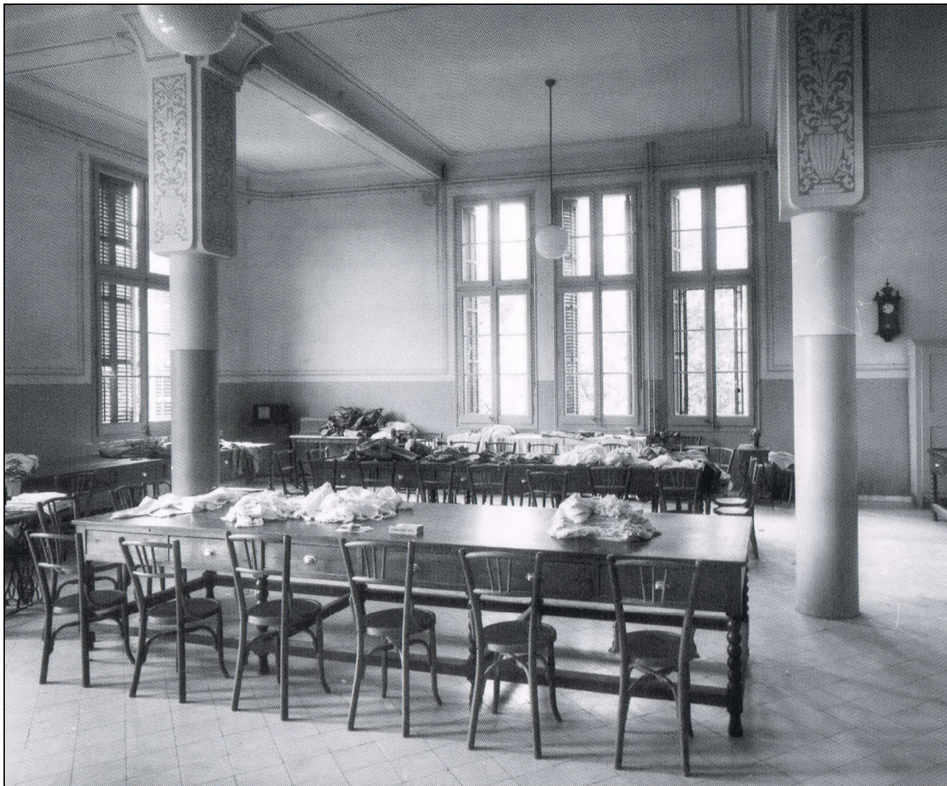
South side room of ground floor in pavilion Rosa
