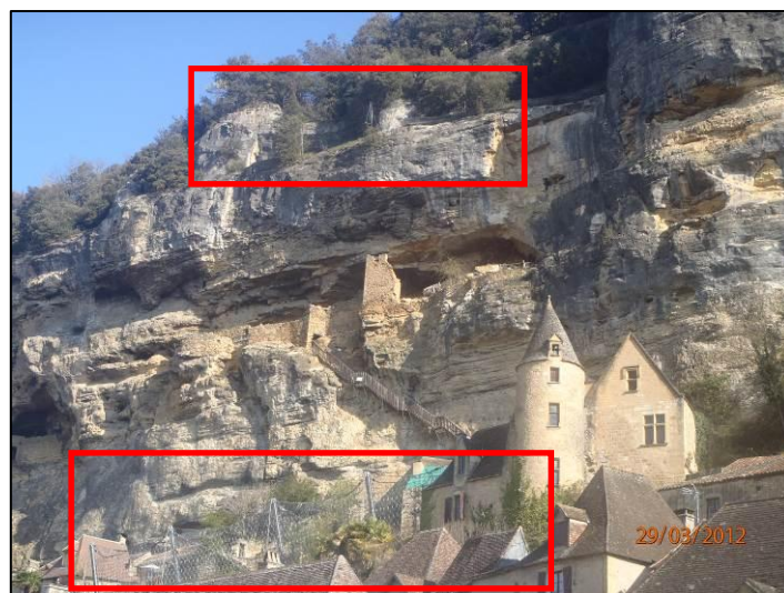
Figure 2-12. Mesh for smalls to medium rockfalls
