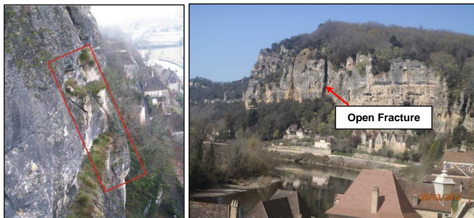
Figure 2-16. Open fractures and decompressed zones of another cliff near to site of study.
