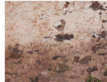
Fig.61. Plastered over the wall
