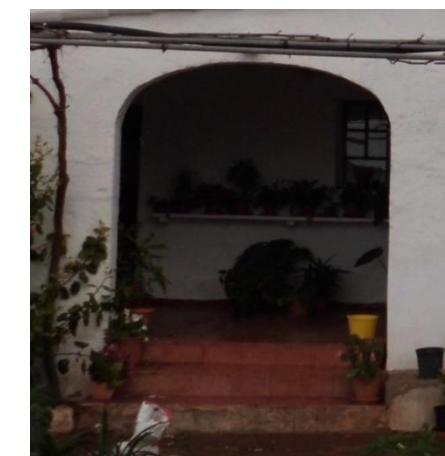
Fig. 21. Example of a survey from the building 1 bow
