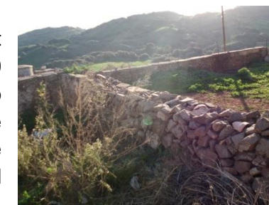
Fig.17. Dry Stone wall
