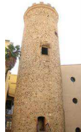
Tower of the palace: current image
