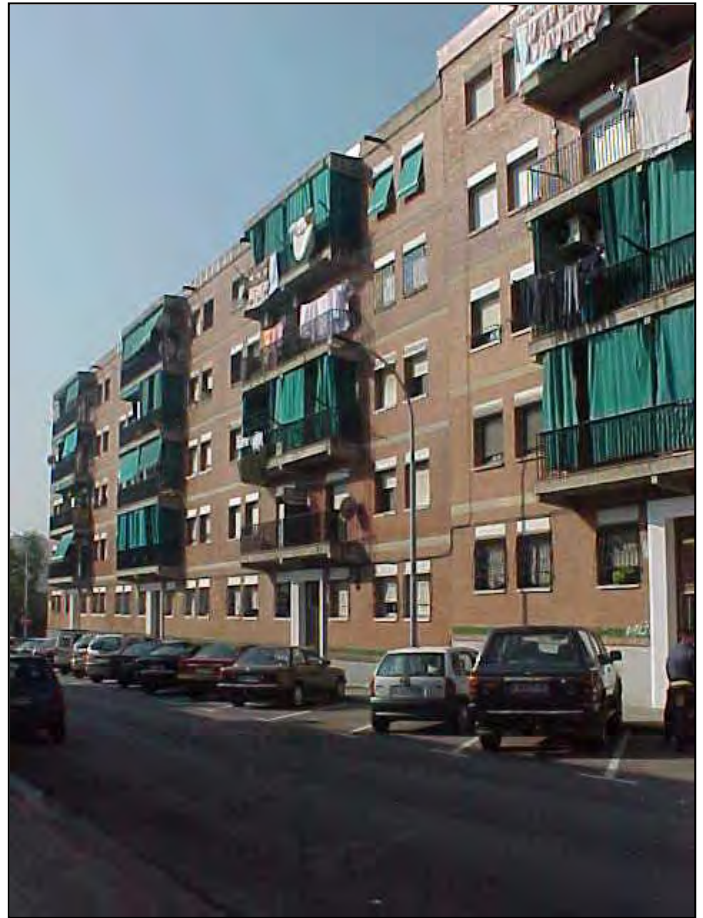
Façana principal Vista general
