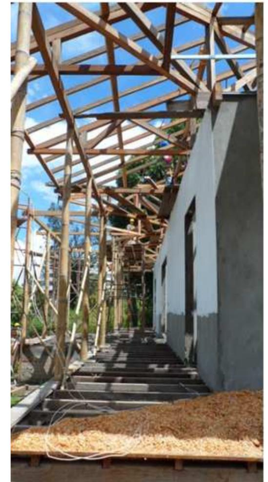
Figure 3.24. Cemented bahareque construction, La Alhambra, Manizales. Personal document.
