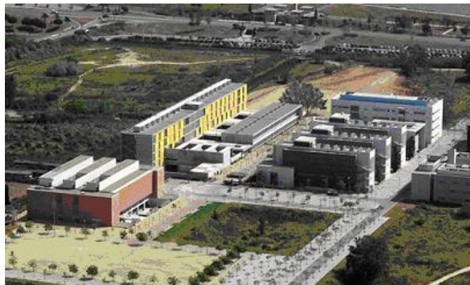
Fig. 3.1. Aerial view of the campus [2]
