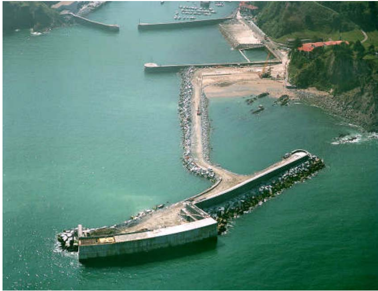
Figure 2.8: Aerial picture of the breakwater integrated OWC plant in Mutriku, Basque Country, Spain.
