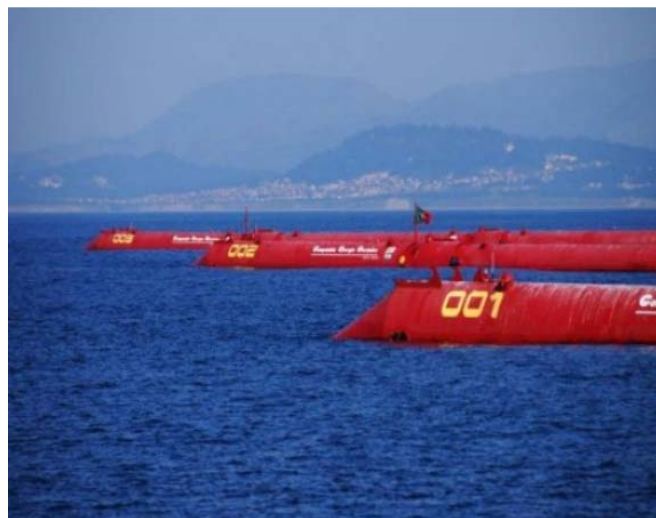
Figure 2.14: Different Pictures of the Pelamis device. The first picture shows the prototype in a front view while it was being tested in the English coasts. The Second shows how it was introduced into the water. The third pictures shows the wave energy plant that was installed in the Portuguese coast, composed by three devices.
