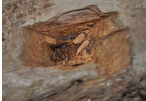
Illustration 22: Extraction hole of a rusty nail
