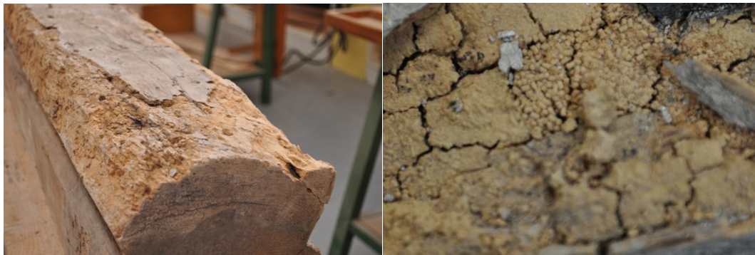
Illustration 20: Galleries, sciure and Hylotrupes bajulus droppings
