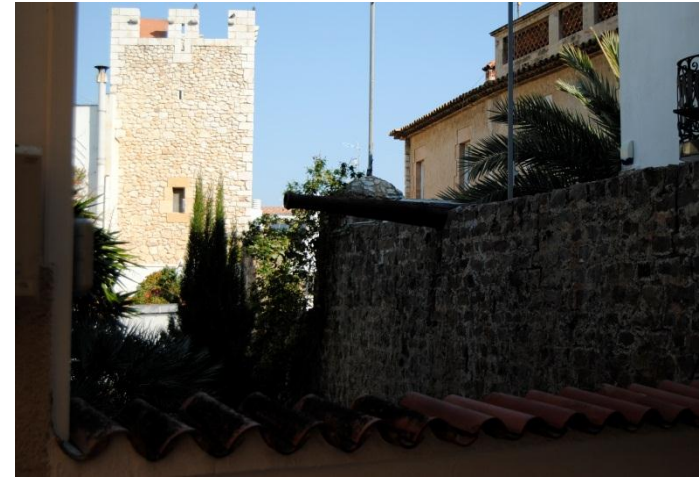
2.4. Part of the expansion of the wall with the Palau del Rei Moro in the background.
