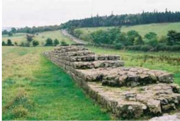
Figure 1 Hadrian's Wall, England, a few miles east of Housesteads was built in A.D. 122 by three Roman Legions, using local materials available, and in some parts the stone faced an inner core composed of concrete and rubble (Source: www.understandin-cement.com ).
