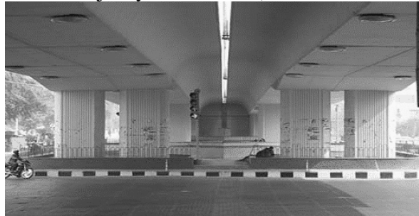
Figura 2.7. Kalkaji Flyover, Delhi ( www.theconstructor.org )
