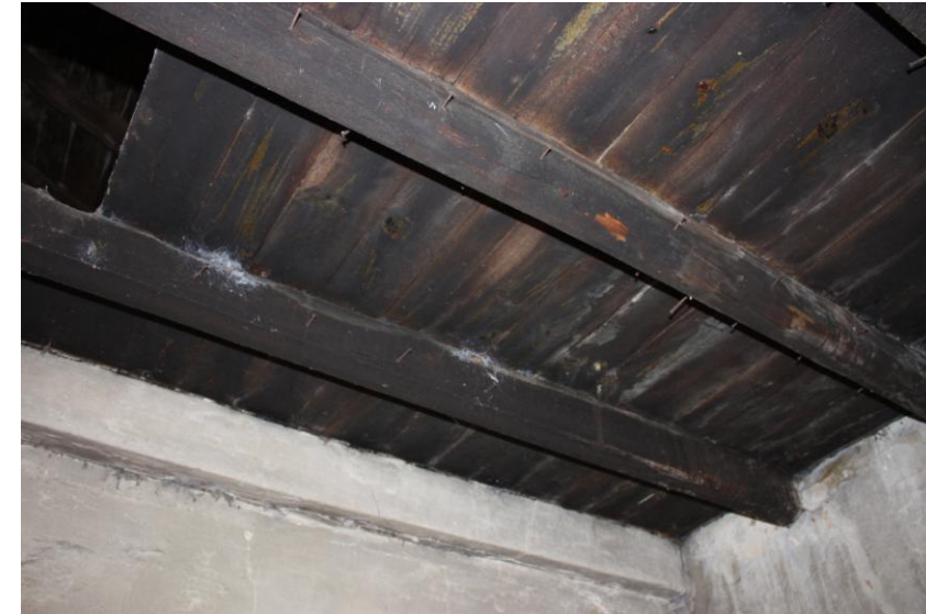
11.- False ceiling with wooden boards.
