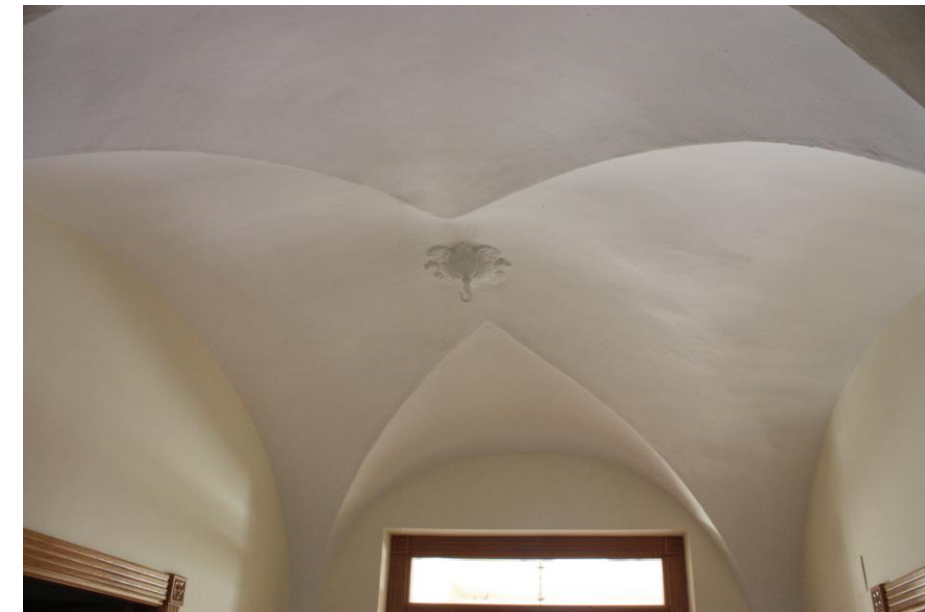
9.- Solid brick coated vault.
