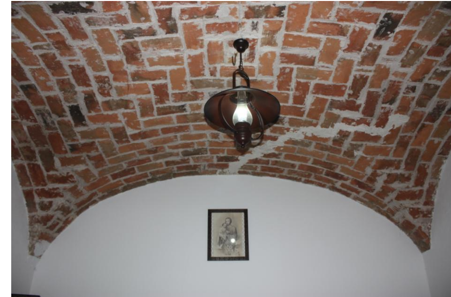
8.- Solid brick vault uncoated.
