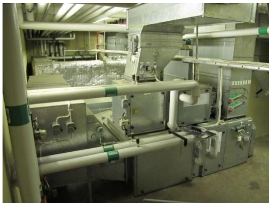
Figure 45: Aggregate room B59
