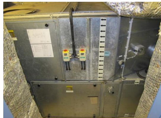
Figure 46: Aggregate room B33
