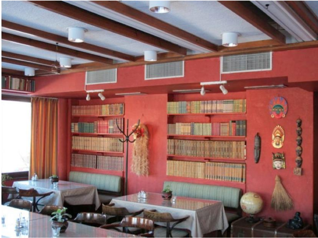
Figure 53: Example of mixing ventilation 2
