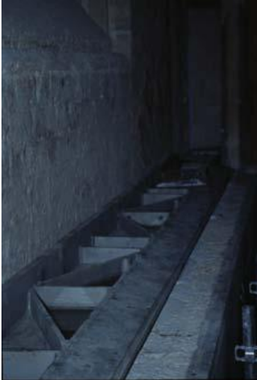
Figure 6.5.8 The trussed steel beams placed over the cornice inside the Basilica
