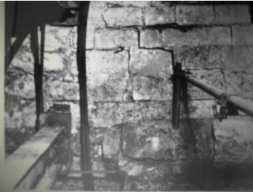
Figure 6.9.4 North-east pier foundation, York Minster, England
