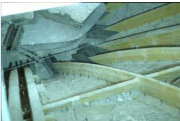
Figure 6.5.10 The ribs covered with aramidic fiber tissue Figure 6.5.11 The tie bars and springs
