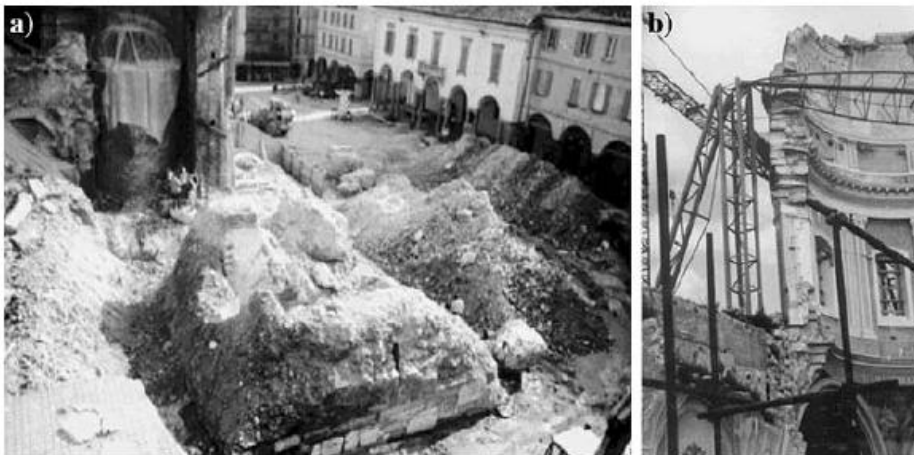
Figure 5.2.5.4 Collapse of Civic Tower of Pavia (1989) (a) and Cathedral of Noto (Siracusa, 1996) (b), Italy
