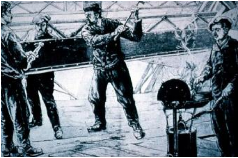
Figure I.5 The change from cast iron, with elements that fitted together, to wrought iron, joined by rivets, had a significant effect on the appearance of joints.
