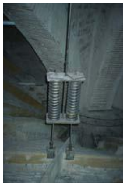
Figure 6.5.10 The ribs covered with aramidic fiber tissue Figure 6.5.11 The tie bars and springs
