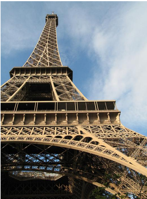
Figure I. 1 The Eiffel tower is constructed from puddle iron, a form of wrought iron.
