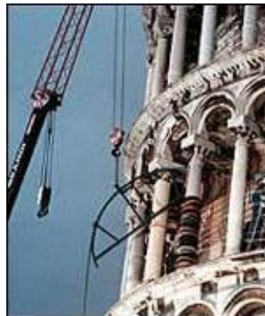
Figure 6.4.6 A steel corset was placed around the tower
