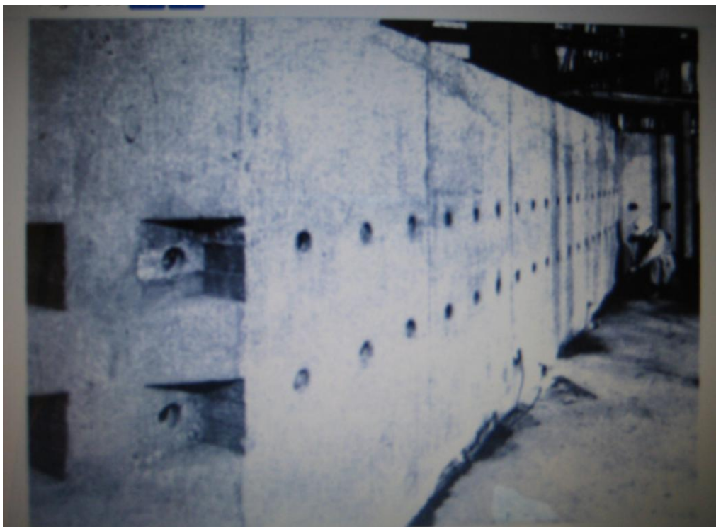
Figure 5.3.7.2. Enlarged foundations, central tower, York Minster, England
