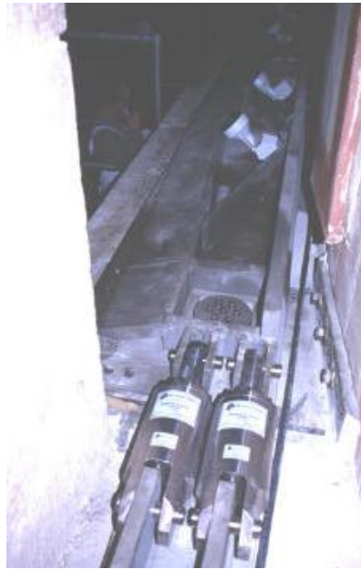
Figure 6.5.4 The three sets of installed SMADs Figure 6.5.5 The installed STUs.
