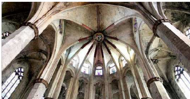
Figure 2.15 – Vault with palm shape in altar
