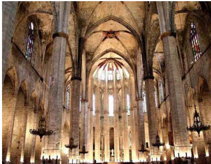
Figure 2.2 - Internal view of the church
