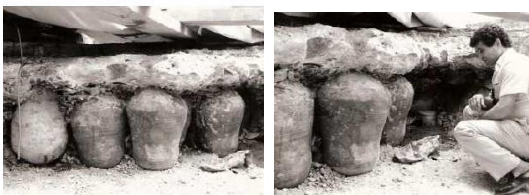
Figure 2.26 - Infill of the central vault (pictures done in the 1990s)
