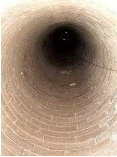
Figure 2.27 Central empty space and internal wall of the tower
