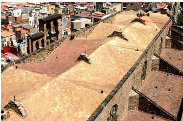
Figure 2.12 – View of the roof of the central nave
