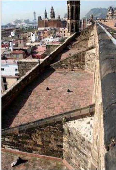
Figure 2.10 – View of the roof of the lateral nave
