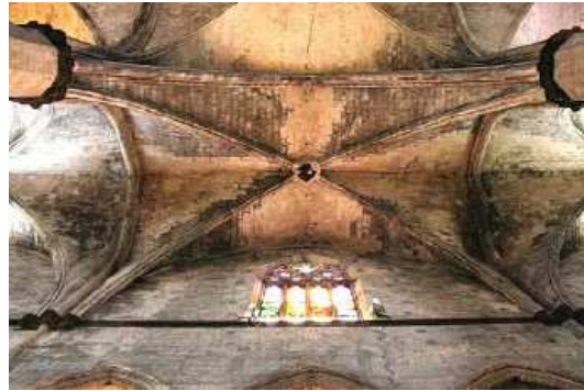
Figure 2.14 – Rectangular cross vault at lateral nave
