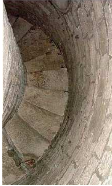
Figure 2.28 – Stairs space between internal and external wall
