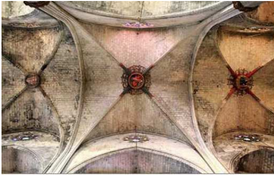
Figure 2.13 – Square cross vault at central nave
