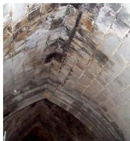
Figure 2.37– Relative displacement in arch and vault key
