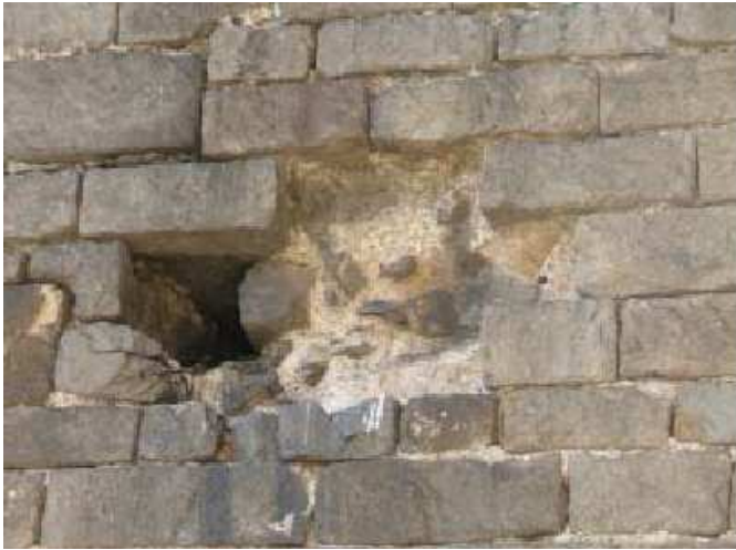
Figure 2.22 Hole in the wall (interior composition visible)
