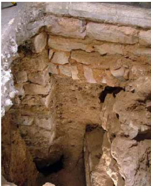
Figure 2.20 Buttress Foundation at the head of the church
