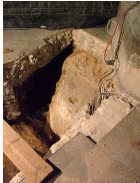
Figure 2.21 – Pier foundation
