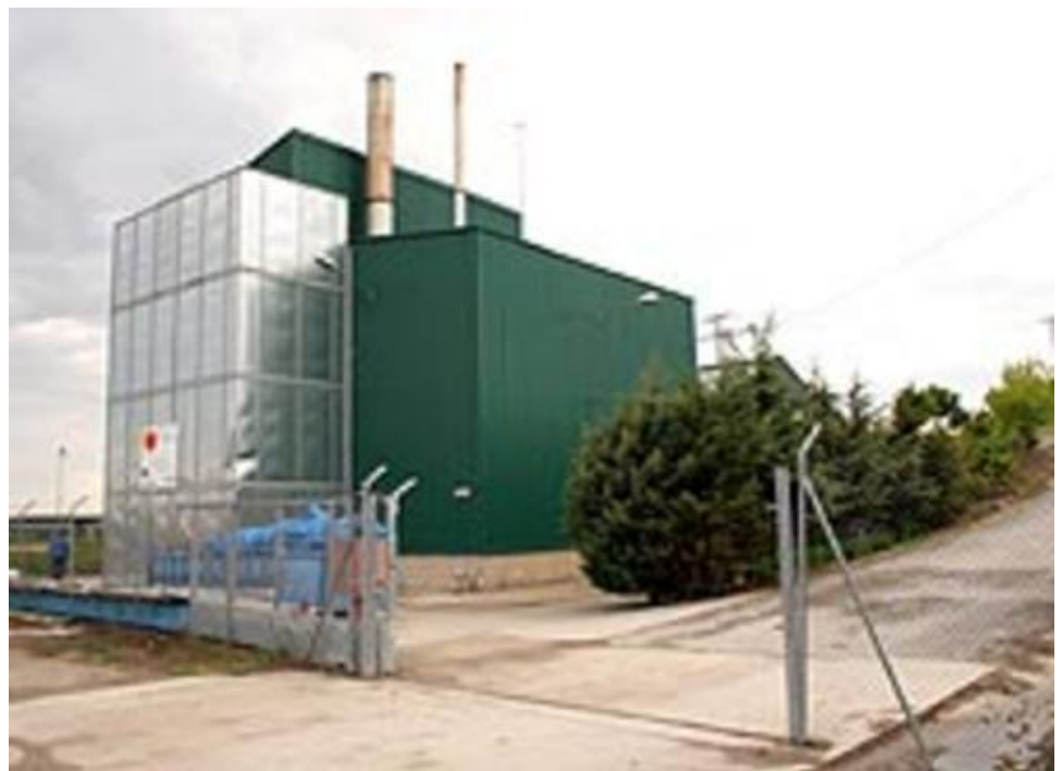
FIGURE 22. Biomass plant located in Cuellar, Segovia. Source: http://habitat.aq.upm.es/bpes/onu00/bp347.html
