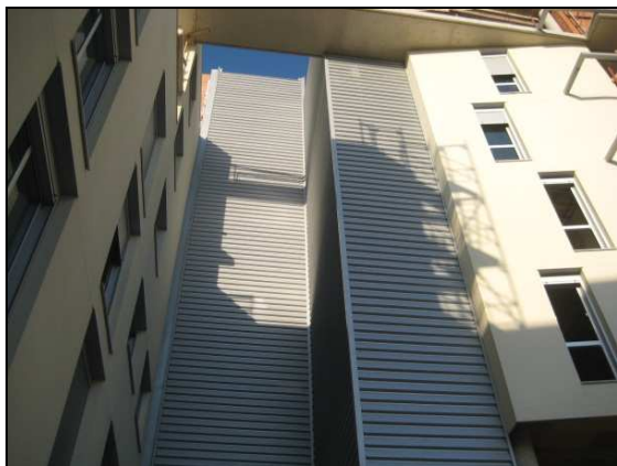
Foto 4.18: Tancaments Embastiata exterior
