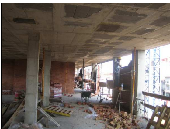
Foto 4.15: Tancaments vista interior
