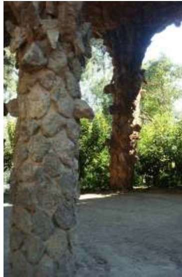
Figure 3.16 The main columns of the north and south side of the lower viaduct are alternating rather than opposing each other
