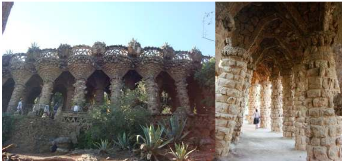
Figure 3.7 Left: View of the upper viaduct Right: Bearing structure of the upper viaduct
