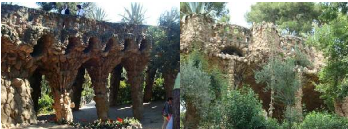
Figure 3.12 Left: General view from the north side of the lower viaduct Right: General view from the south side
