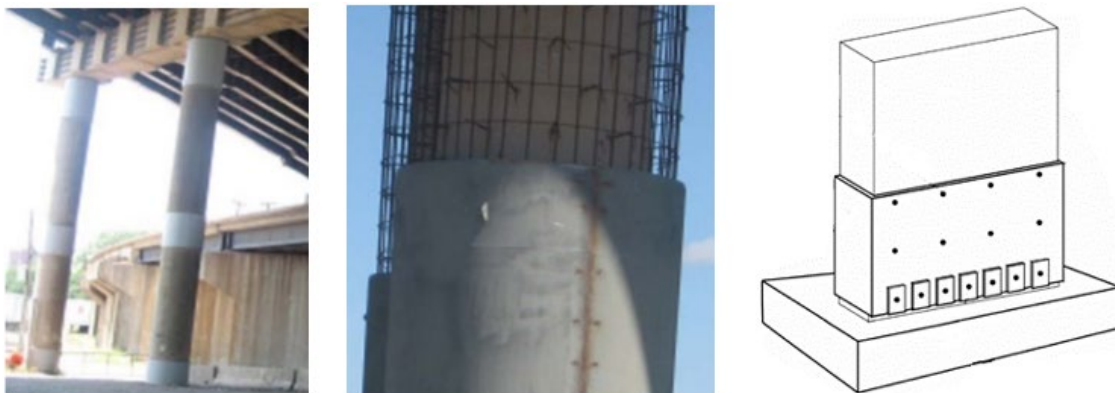
Figure E.4 Jackets from Left to Right: Steel Jackets, Concrete Overlays, and Steel Plate Encasement with Steel Anchors (Buckle, Friedland, et al., 2006; Timothy et al., 2011)
