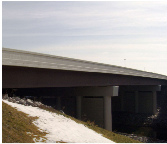
Figure D.54 Pier Detail from Inspection Photos (NBI 50795) (BIAS)
