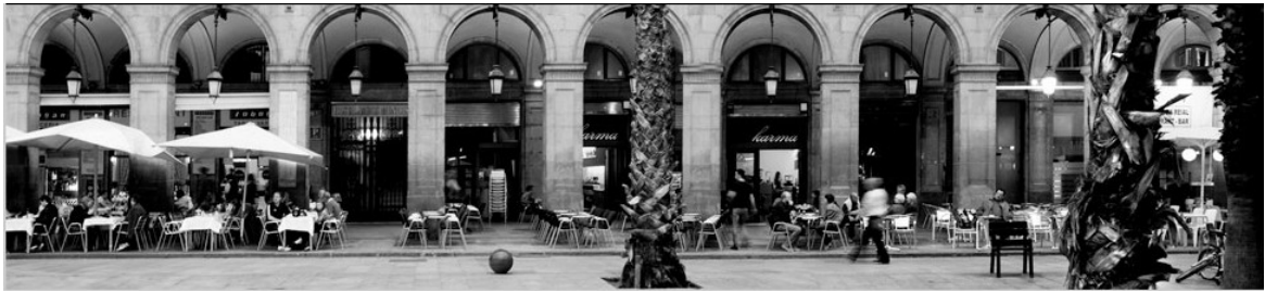
Fig. 54 – Façade with series of arches in the Plaça Reial. (La Plaça Reial)
