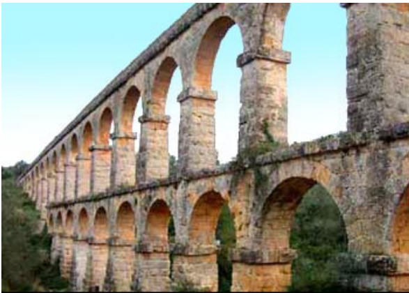
Fig. 75 – Aqueduct of Las Ferreras in Tarragona (The History of the Spanish Architecture)
