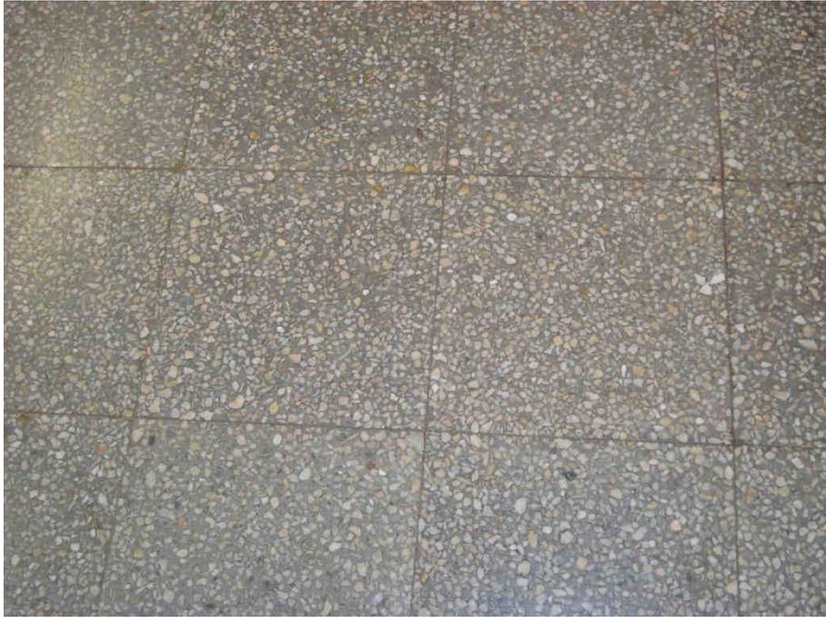
This is stone tile floor artificial. Its dimensions are 40 x 40 cm. This floor is on the stairs.
