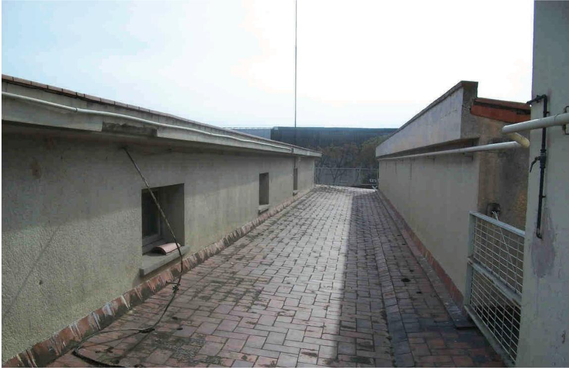
*In this picture you can see the two types of roofs. To the right is the cover ventilated and on the left is the slab concrete cover.*
