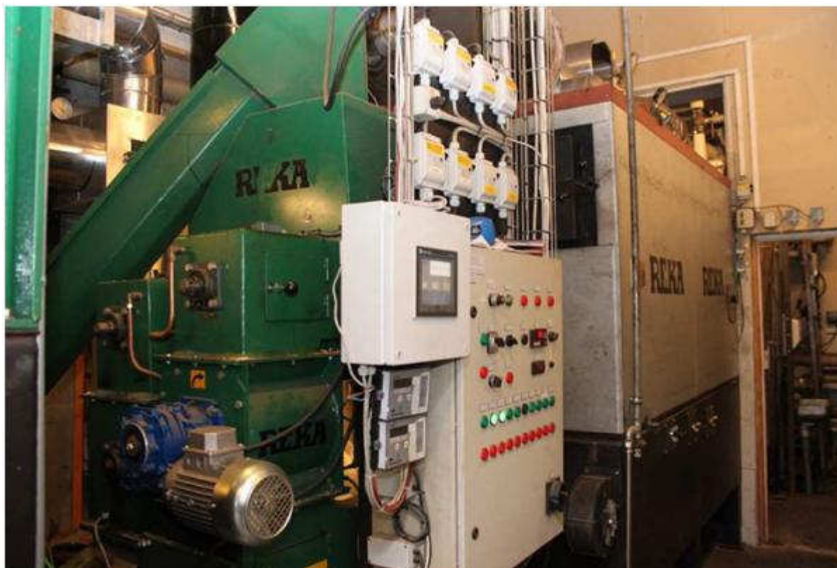
Picture 4.4.3: Later on, they installed a central wood chip stove (160kW):
