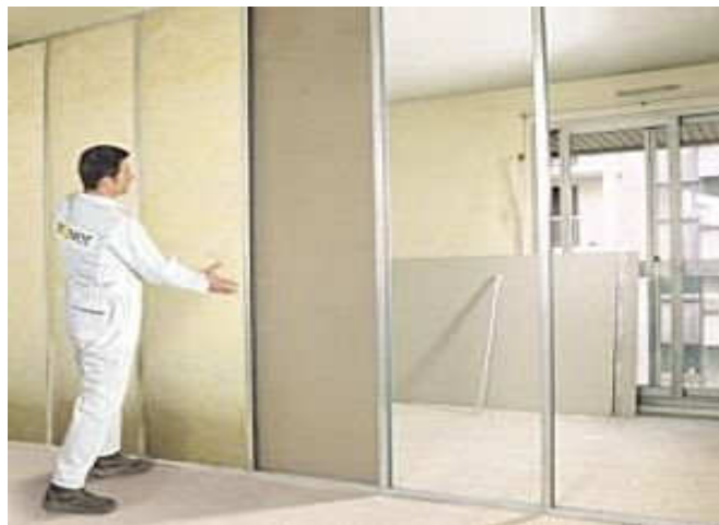
Figure 6.1.1. Installation of wall insulation. http://www.placo.fr
