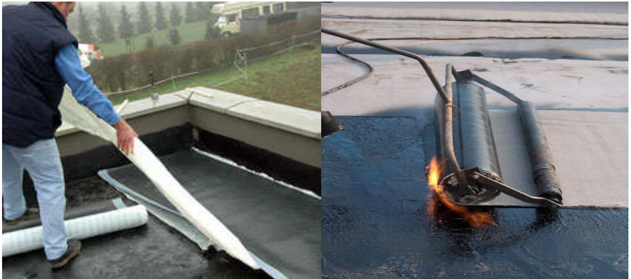
Figure 6.1.3. Installation of roof sealing. http://www.barbot-guesdon.fr
