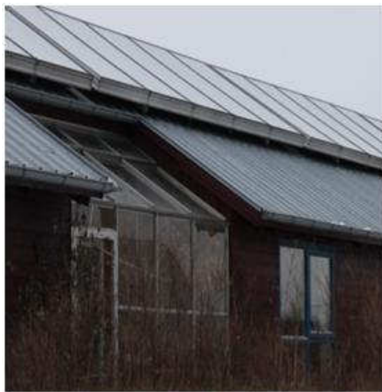
Picture 4.4.8: Roof of the house
