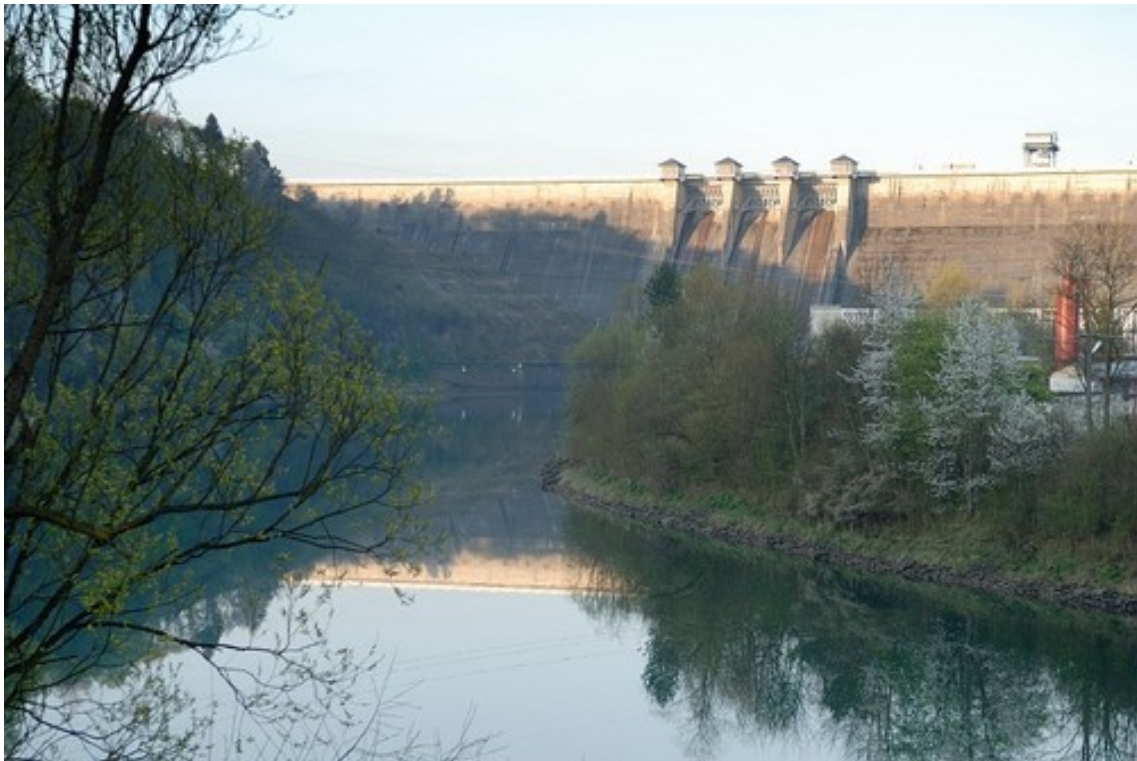
Figure 71. The dam on Solina lake, Panoramio 2008.
