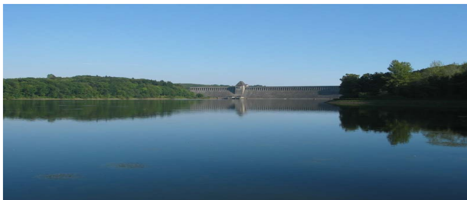
Figure 80. The dam of the Möhne reservoir, Wikipedia 2008.
