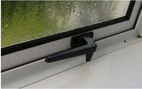
Figure 9. Water condensation, Thermalframe PCVu 2008.
