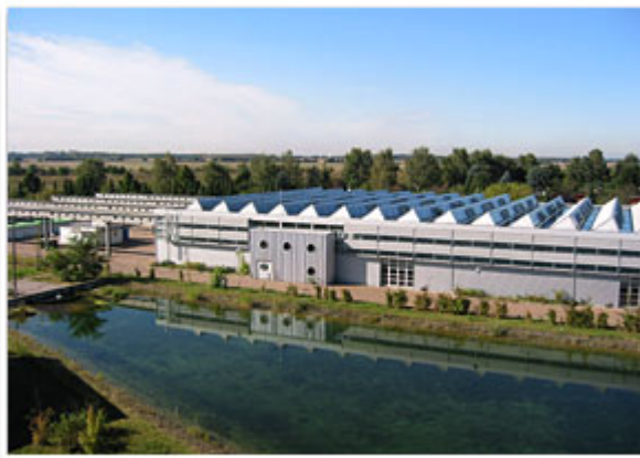
Figure 81. View of the hall housing the indoor artificial ponds, Umweltbundesamt 2008.
