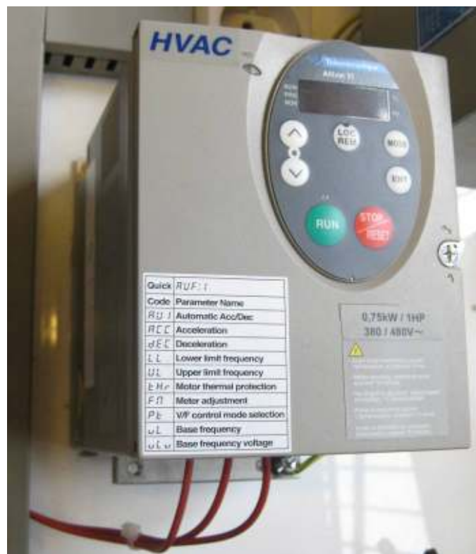
Figure 7.3. Photo of variable speed drives practice.
