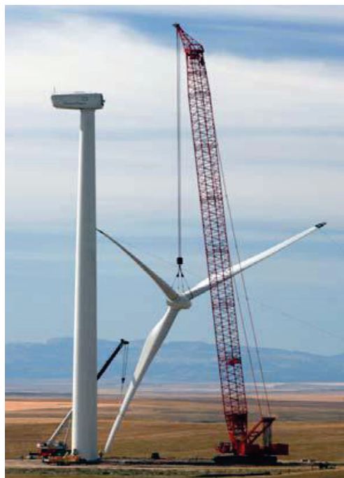
Figure 8.3: Mounting a wind turbine
