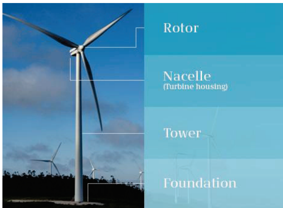
Figure 8.1: the different part of the wind turbine (source: Vestas website)
