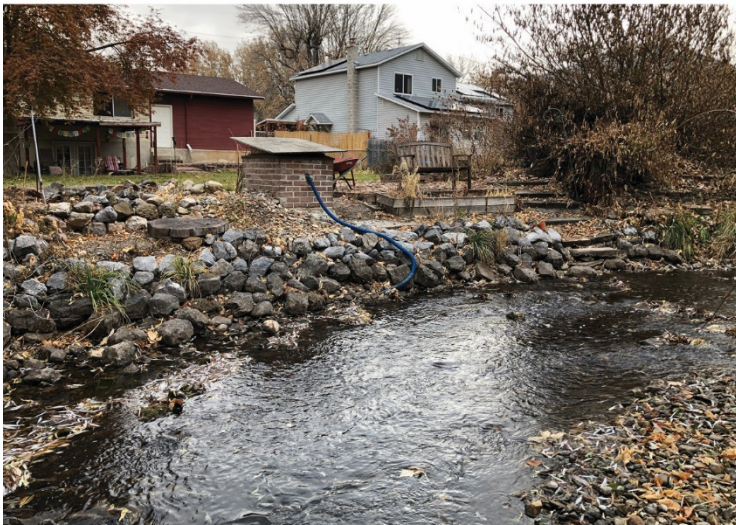
K - Backyard pump across from Jens Johansen Park
