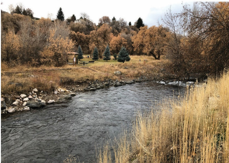
I - Left bank at Denzil Stewart Nature Park. Some erosion
