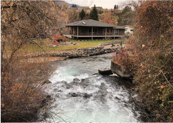
M - Looking down the spillway from the Crockett canal
