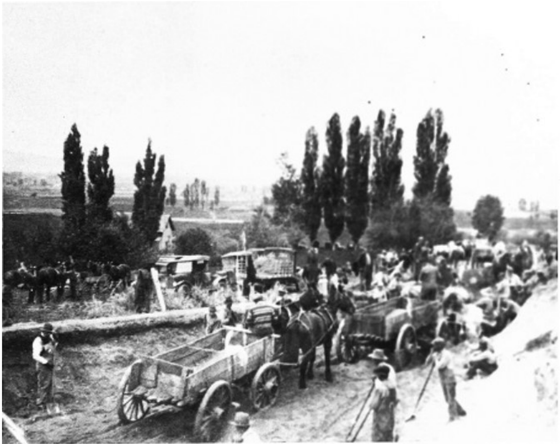
Figure 31. Digging the Logan Northern Canal.
