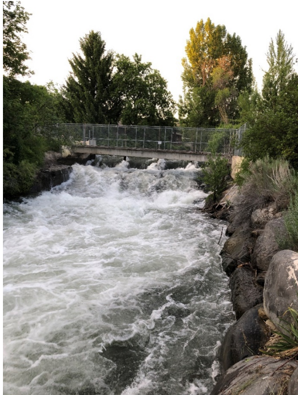
Figure 4. Pedestrian Bridge over Crockett Diversion
