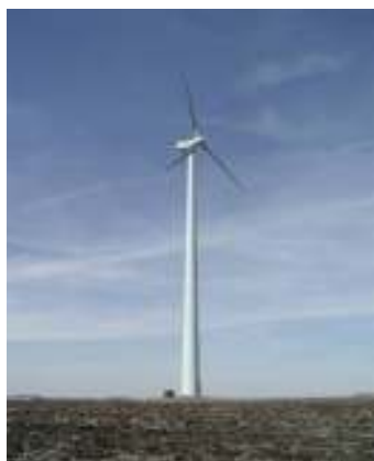
Figure 3.1.4 Tubular steel towers.
