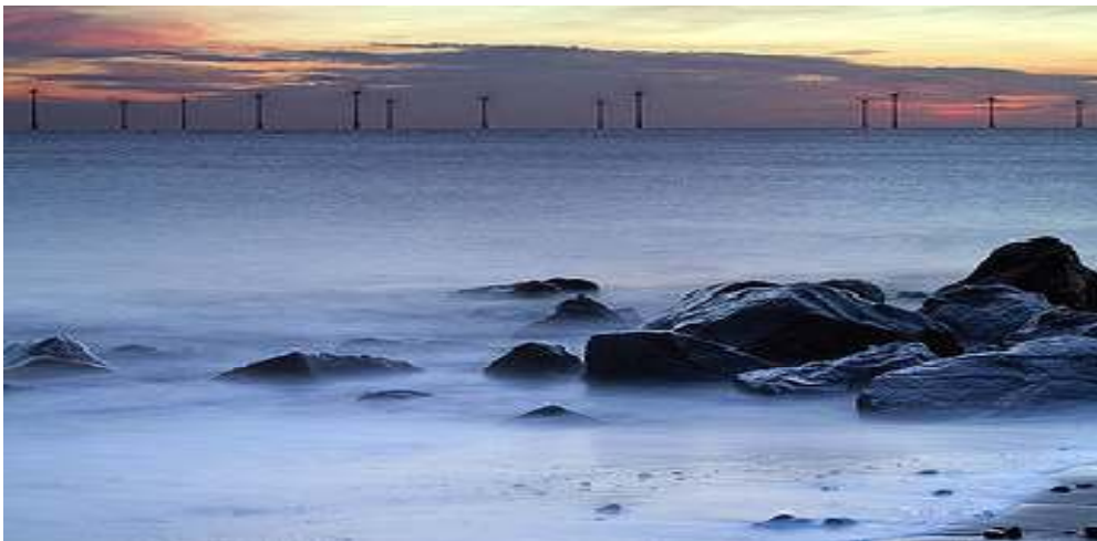
Figure 4.2.2 Scroby Sands seen from the beach. The distance is 2.5 km with turbines of 2 MW, 80 m of diameter and the nacelle high is 60 m. As it can be seen in this picture the visual impact is important.
