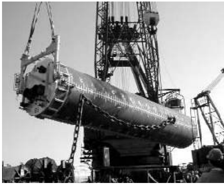
Figure 4.3.12: Suction caissons for an offshore platform being transported to site in the Gulf of Mexico. (Courtesy of E. C. Clukey).
