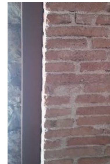
Picture 3.14: artificial stone plinth. Muntaner, 178. Source: Own made.
