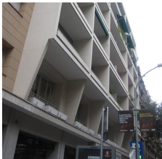
Picture 3.30: Fixed solar protection, horizontal projecture. Some apartments also have an added mobile protection, awning. Rosselló, 214. Source: Own made.
