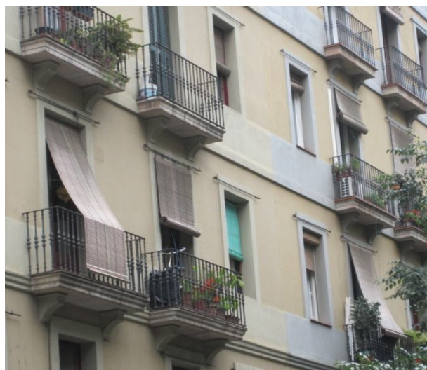
Picture 3.38: Rope shutter. Consell de Cent, 222. Source: Own made.
