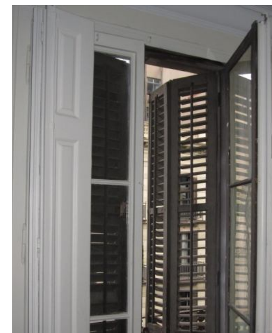
Picture 3.34: Window with slat solar protection and a interior "contrafinestra". València 261. Source: Own made.
