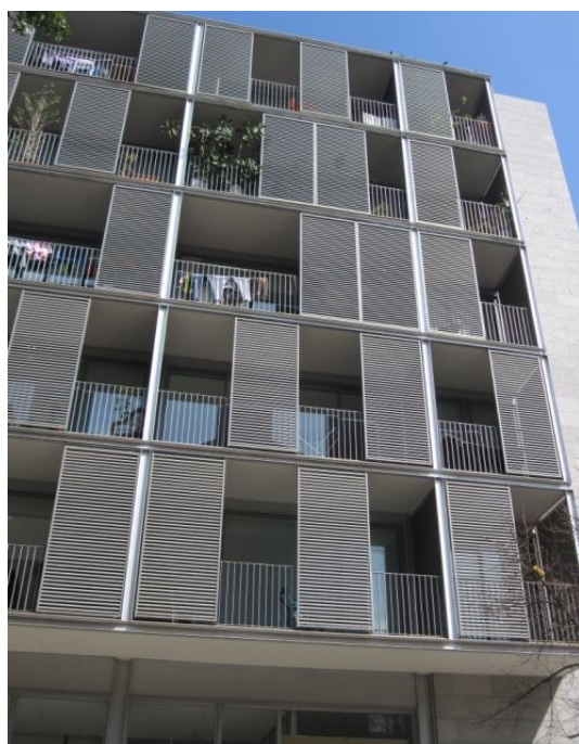
Picture 3.31: Lateral concealeable solar protection. Ali Bei, 57. Source: Own made.
