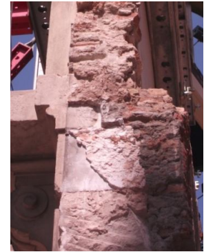
Picture 3.1: Difference in thickness between the ground floor facade and types facade. Còrsega, 294. Source: Own made.
