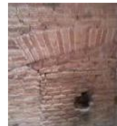
Picture 3.15: Back with brickwork. Consell de Cent No. 377. Source: Own made.
