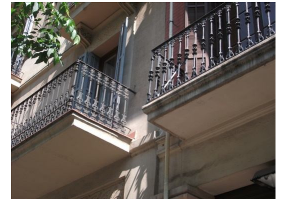
Picture 3.26: Projectures balconies over 70cm. Rosselló, 156-158. Source: Own made.
