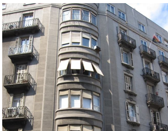
Figura 3.32: Vertical concealeable solar protection. Consell de Cent, 413-415. Source: Own made.
