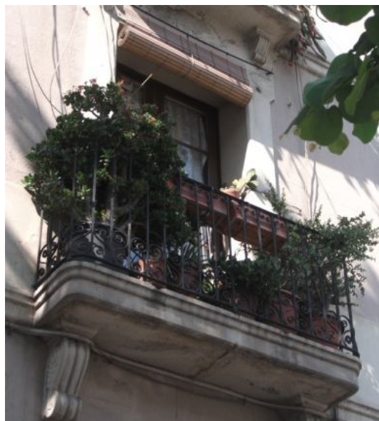
Picture 3.25: Balcony overhang of 40 cm. Source: Own.
