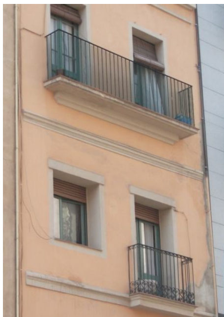
Picture 3.20: continuous coating layer. Rosselló, 147. Source: Own made.
