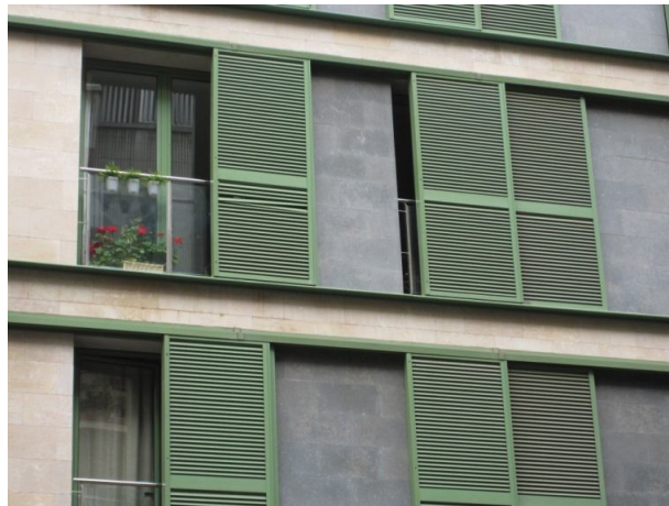
Picture 3.37: Lateral sliding shutter. Calàbria, 178-180. Source: Own made.
