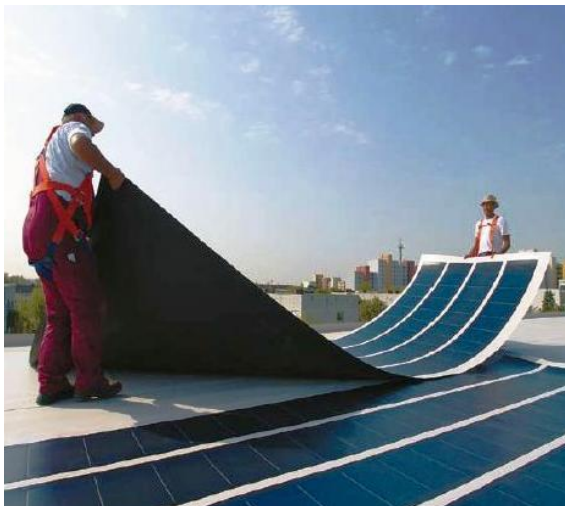
Figure 12.4. Flexible solar panels using organic solar cells, by WILEY-VCH
