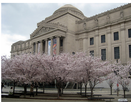
Figure 2 The Brooklyn Museum, a masonry clad steel-framed building, was built in 1897 (NY,USA)
