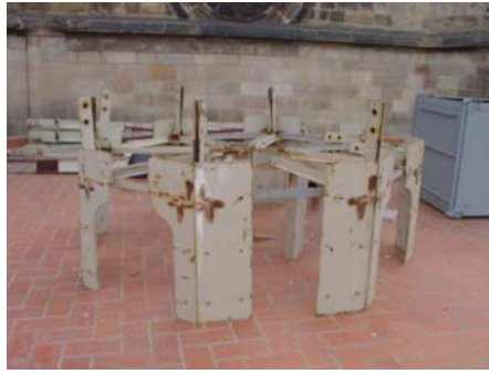
Figure 22 The support of the dome.
