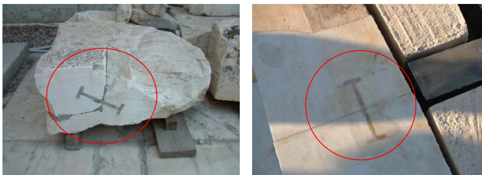
Figure 13 Modern use of titanium to replace steel strengthening
