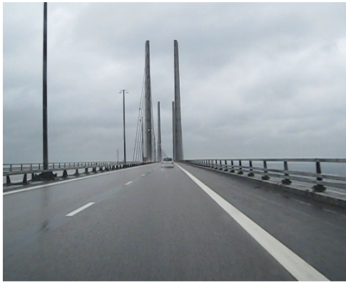
(a) Measurement location: Bridge
