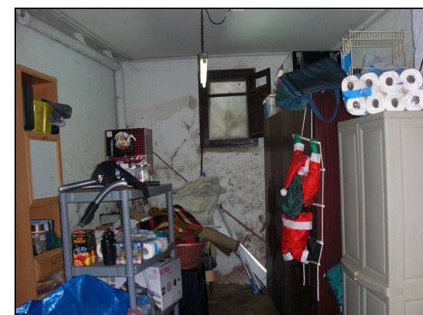
Fig. 3.11 Bodega - Safareig. Vista 1
