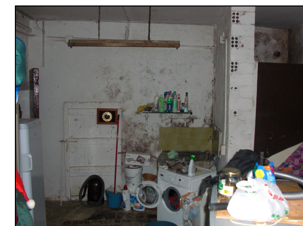
Fig. 3.12 Bodega - Safareig. Vista 2
