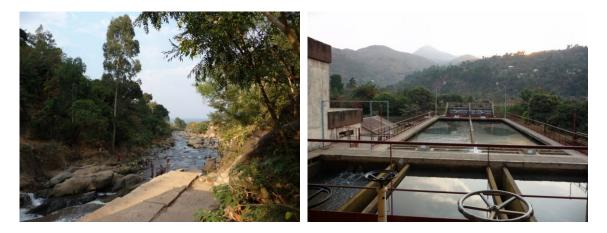
Figure 2-10 Water intake chamber on the river Mulongwe (left) and decantation reservoirs at the water treatment station (right)
