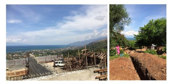
Figure 2-12 Construction of a new reservoir on the hills of Kiyaya overlooking northern Uvira (left); new water pipes being laid in Kasenga neighbourhood (right)
