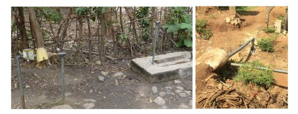
Figure 2-11 Typical tap connection with the tap protected by a lock and meter by a plastic cover (left); exposed water pipe following soil erosion (right)
