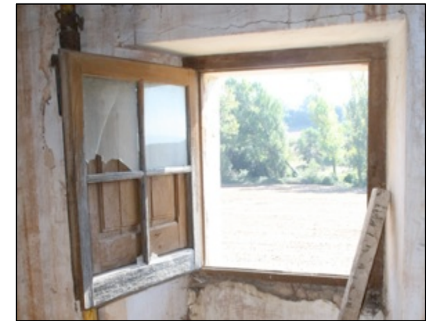
Photo 6: First floor Hall 1 window
