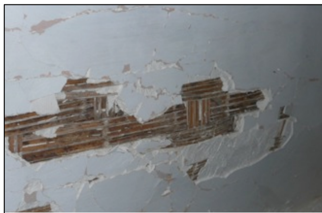
Photo 10: First floor rooms false ceiling
