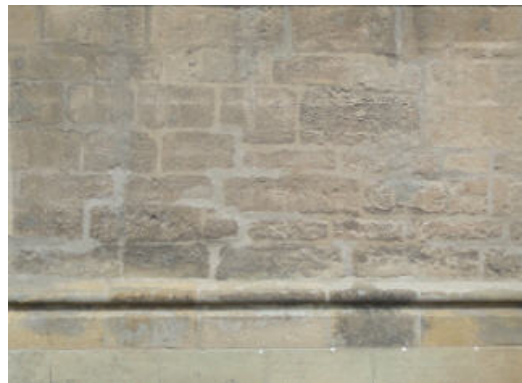
Figure 21 Repointing on the exterior walls
