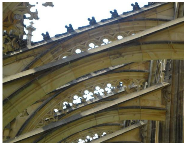
Figure 26 Strengthened flying arches
