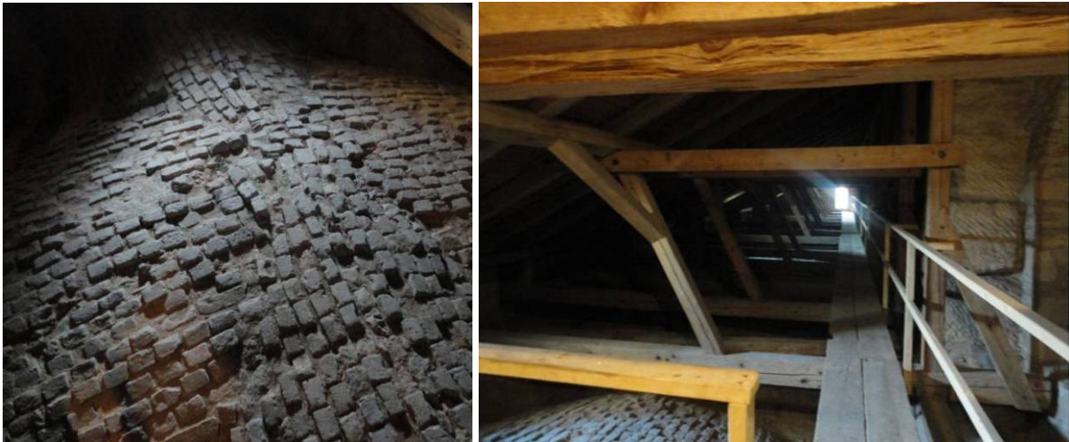
Figure 41 a) Extrados of the vaults b) Timber structure from the roof
