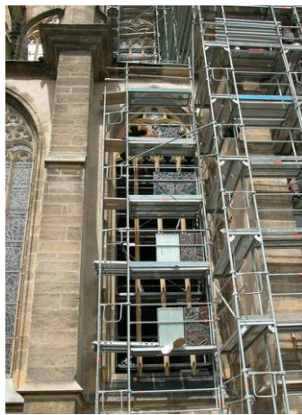
Figure 20 Restoration of the stained windows [13]
