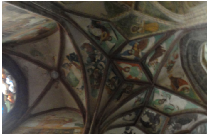
Figure 32 Vault of the ambulatory and chapels
