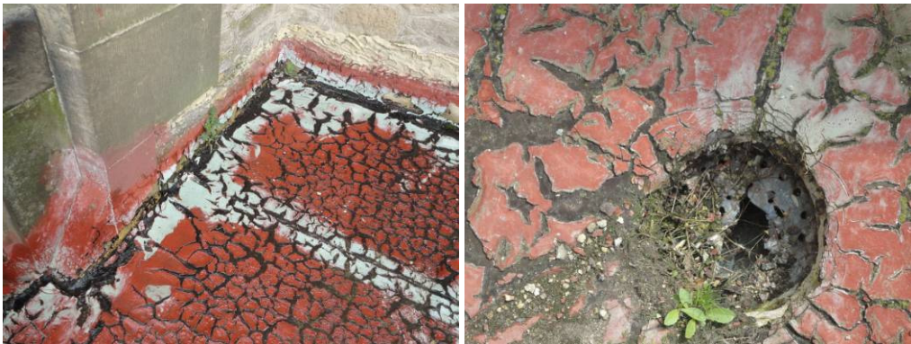
Figure 23 Asphalt layers of the balcony floor
