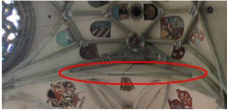
Figure 35 Railway rail located between the vaults
