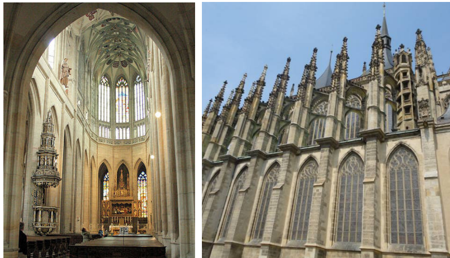
Figure 13 a) Interior east view b) Exterior south view
