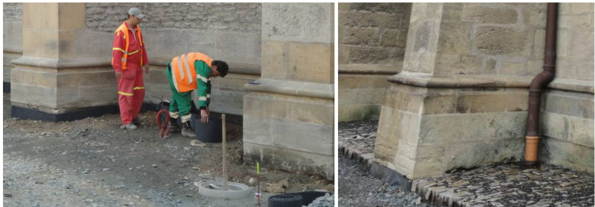
Figure 30 Geotextile and porous fill
