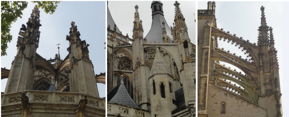
Figure 25 Type of Buttresses
