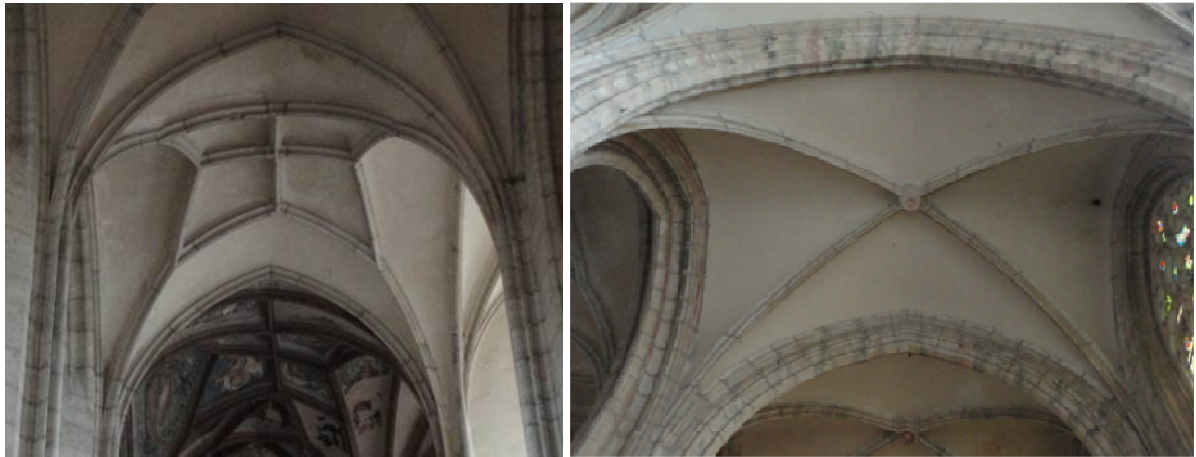
Figure 33 a) Vault of the aisle b) Vault of the lateral naves
