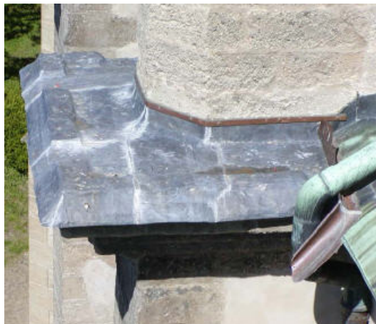
Figure 42 Lead flashing on a cornice
