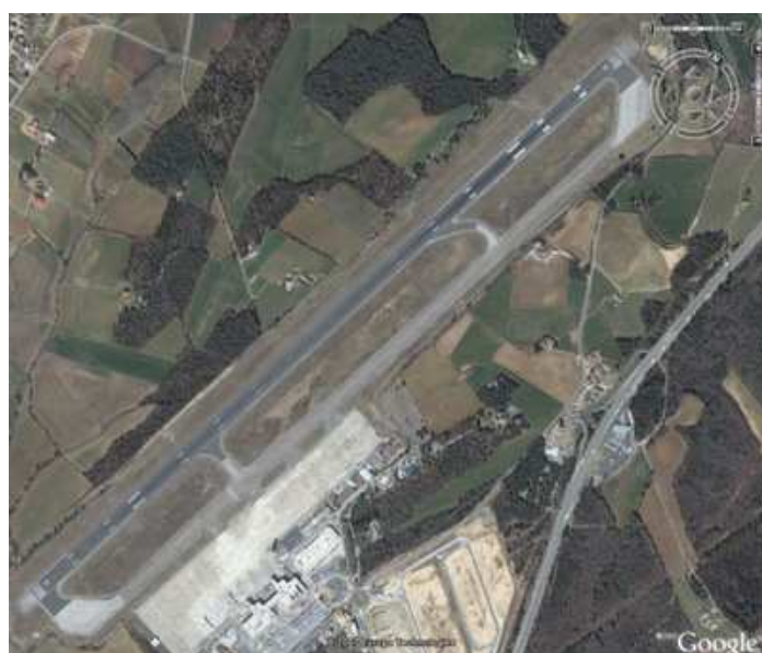
Figure 7.5. Girona–Costa Brava airport [W6]
