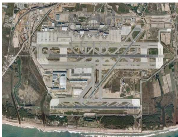
Figure 12.10. Barcelona Airport in 2009 (T1 terminal construction) [S3]
