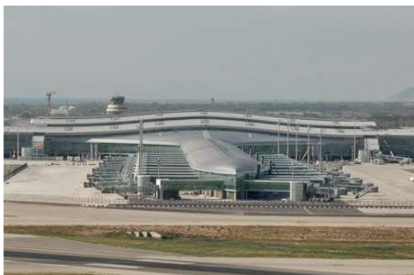
Figure 7.2. Barcelona–El Prat airport T1 Terminal [W8]
