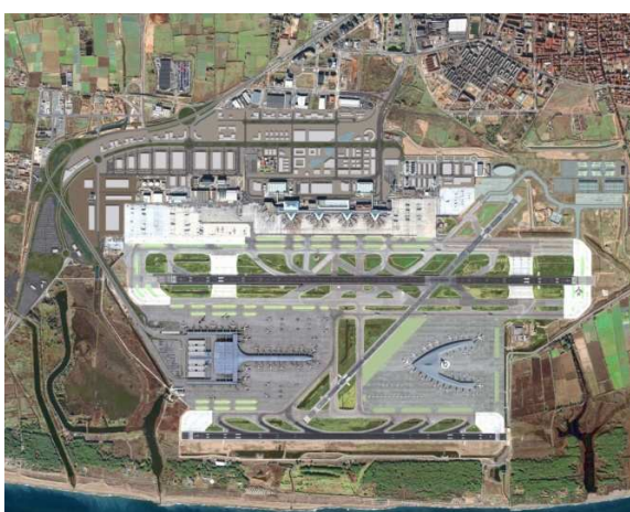
Figure 12.11. Future Barcelona Airport in 2013 (Satellite and Airport city)
