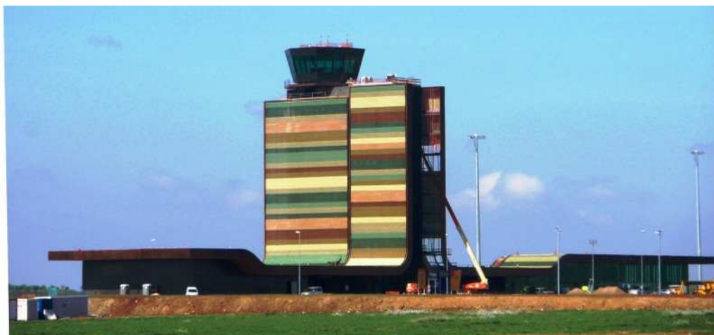
Figure 7.6. Lleida–Alguaire airport Terminal [W11]
