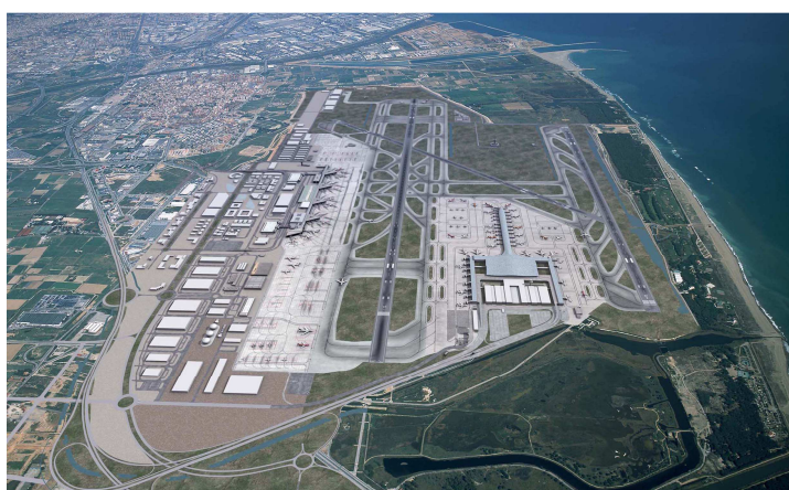
Figure 7.3. Barcelona–El Prat airport [W8]
