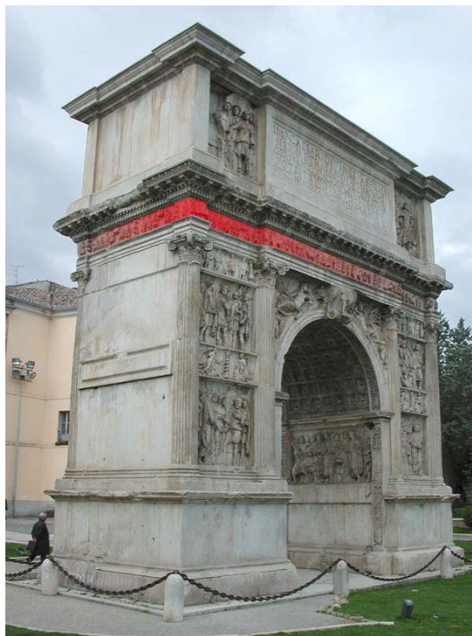
06 – The Traiano Arch minor frieze is 9 mt. high. One of the rapid prototyping purpose is to create a model to allow visitors to have a “closer view” of the ornaments.
