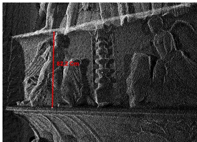
04 – By means of the 3D model it is possible to draw the measures of the architectural elements.
