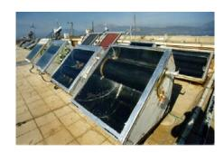
ICS solar water heaters are simpler and aesthetically attractive when integrated in the buildings structure.
