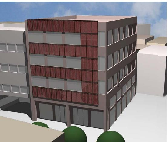
**PV/T** Collectors: The hybrid Photovoltaic/Thermal (PV/T) collectors convert simultaneously solar radiation into electricity and heat, which can be effectively combined with typical thermal collectors. In addition, the booster reflectors are suggested, in order to increase the energy input to collectors.
