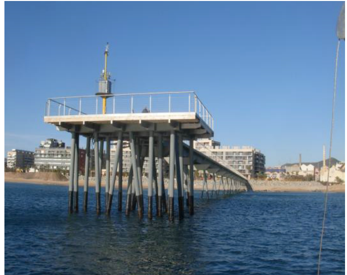
Figure 1 Permanent Pier research station (waves, currents, SSC, temp)
