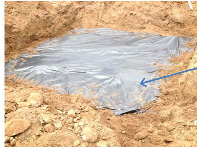
60 mil HDPE hydraulic barrier
