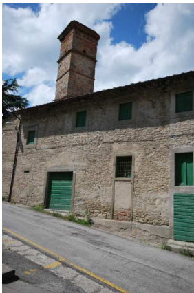
Figure 13 – A small tower within the urban fabric surrounding the Piazza S. Allende in S. Piero in Bagno.
