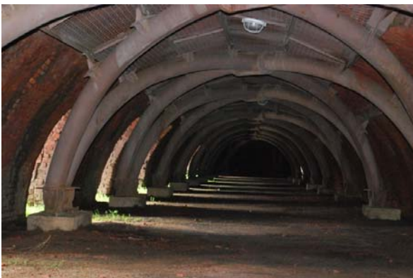
Figure 5 The Interior Chamber of The Hoffman Kiln of Takao (Dagou) Manufactory, Taiwan Tile Corporation (Resource: Author’s Photo)
