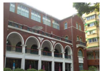
Fig.2: main building (by author)
