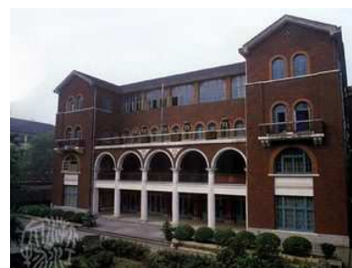
Fig.5: extant main building (by author)
