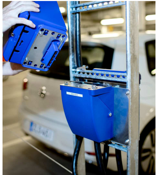
Fig. 1 Example of a charging-ready parking place. It can be converted to a functional charging station by installing the actual charging point through the quick connector [8]
