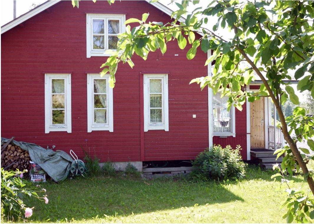
Figure 13. Reuse with traditional style, a form of continued use – not spolia. 1990s summerhouse with older reused windows. Hauho, Finland.
