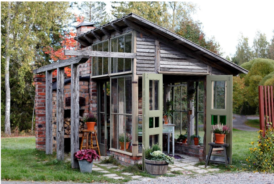
Figure 16. Spolia windows comprising glass curtain walls for a gazebo in Vaasa, Finland.
