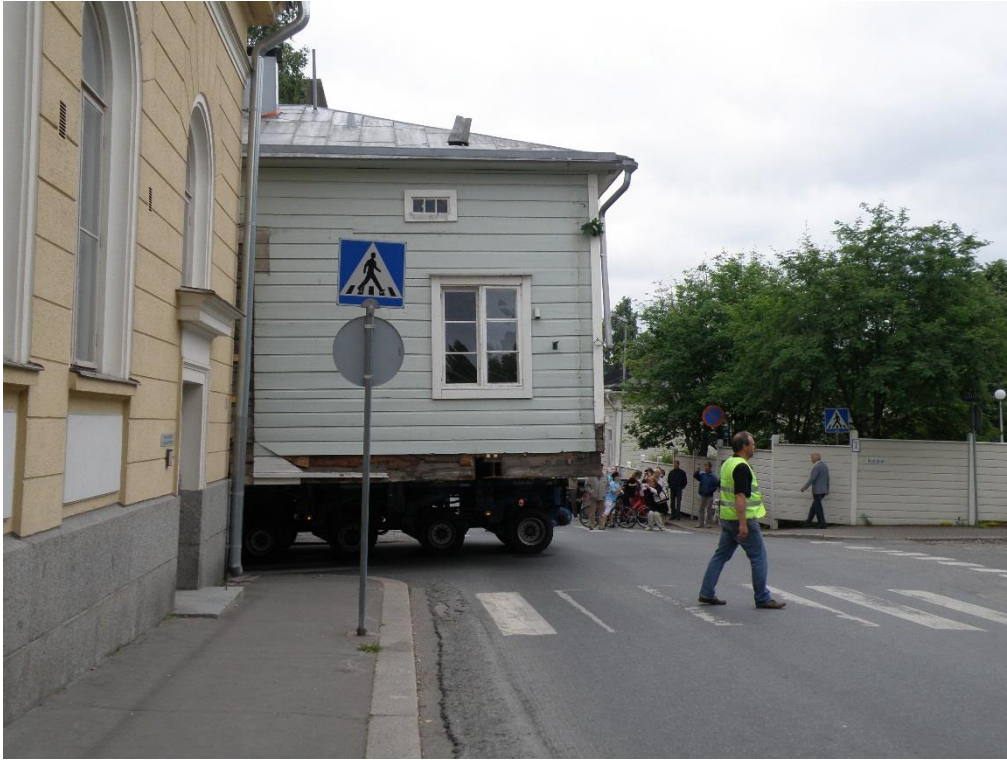
Figure 10. Relocation – not spolia. Moving an entire 19th century house, Hämeenlinna, Finland. Here, the entire building is moved on a lorry but its parts could also have been numbered, deconstructed and reassembled.
