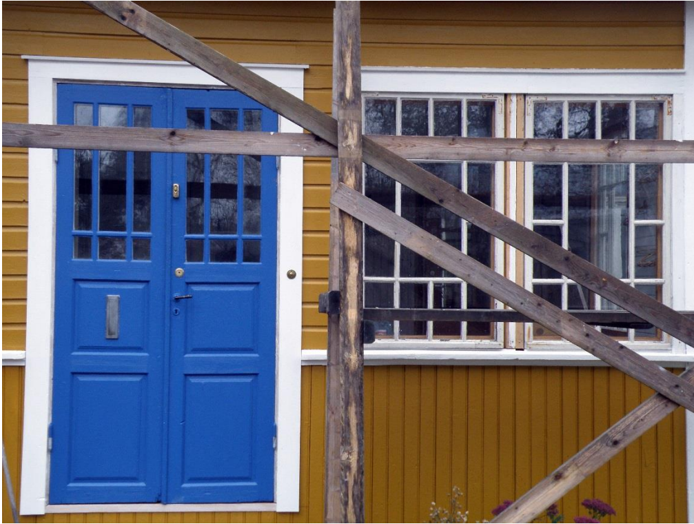
Figure 12. Reuse in restoration, a form of continued use – not spolia. Reclaimed doors double for missing original doors, disposed of without documentation in an earlier renovation. Hämeenlinna, Finland.
