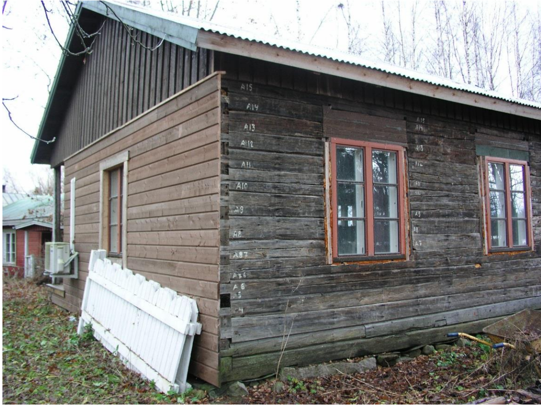
Figure 4. An aged log frame, relocated to its current site in Hauho, Finland, in 2006. The logs are carved to fit the adjoining logs seamlessly; thus they have been numbered prior to deconstruction in order to reassemble them in the same order on the new site. Once the cladding is completed, there is no outwardly visual sign that parts of the building have been relocated.
