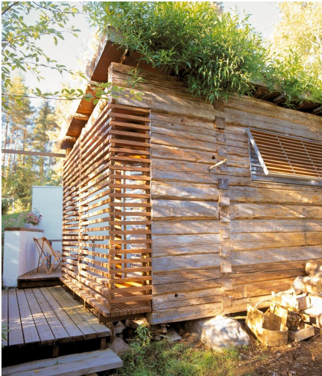
Figure 17. The frame is made of spolia logs but the design does not adhere to the geometry of the original building. Sauna 'Karhi' in Oulu, Finland. The architect is Pave Mikkonen. Photograph courtesy of PAVE Architects.
