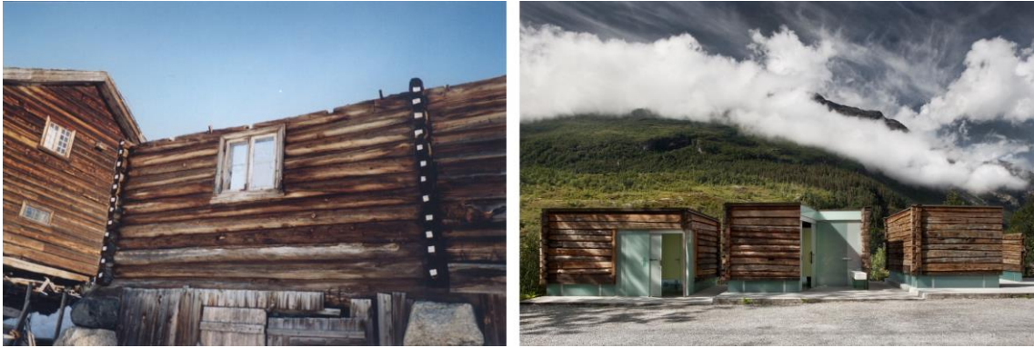
Figure 9. Spolia in timber. The reuse of the log fames of old houses (left) in a contemporary rest-stop (right). Flydalsjuvet, Norway. Right photograph (c) diephotodesigner.de, both images courtesy of 3RW Arkitekter.
