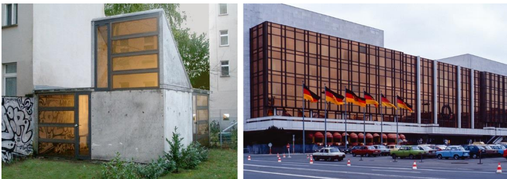
Figure 7. Communicating documentary value to informed viewers. An art gallery in Berlin (left) has very distinguishable spolia windows (photograph courtesy of Wiewiorra Hopp Architekten). The donor building is the GDR's Palace of the Republic (right), demolished in 2006–8 (photograph by Dietmar Rabich, rabich.de, downloaded from Wikimedia Commons and published under the license CC BY-SA 4.0).
