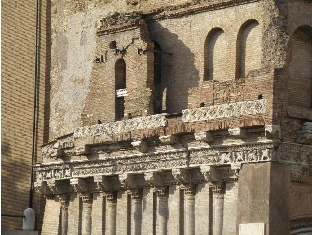
Figure 1. Casa dei Crescenzi (11th century) in Rome is a well-known example of what is traditionally understood by the term, spolia.
