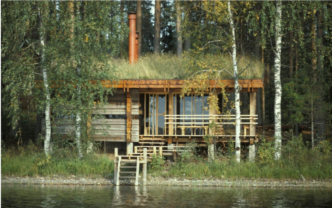
Figure 5. Untraditional, visually prominent reuse of 19th century logs in a 1980s sauna, 'Huitukka' in Juva, Finland. The architect is Georg Grotenfelt. In contemporary Nordic architecture, saunas and summerhouses are typical buildings which can incorporate spolia. Photograph courtesy of the architect.
