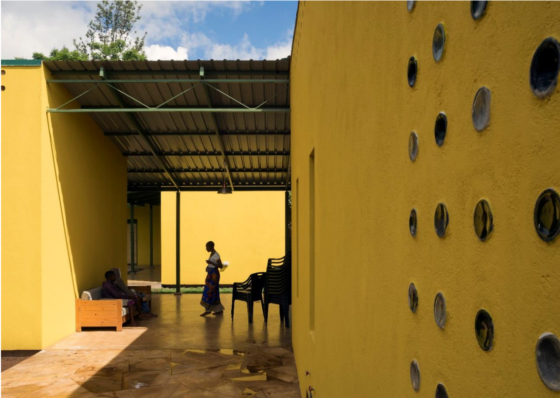
Figure 11. Reuse – not spolia. Glass bottles (right) are everyday commodities, not part of any prior architectural composition. KWIECO refuge, Moshi, Tanzania, designed by Finnish architects Hollmén Reuter Sandman. Photograph by Juha Ilonen, courtesy of the architectural office.
