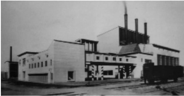
Power house in 1935 (photo by C. Edige)
