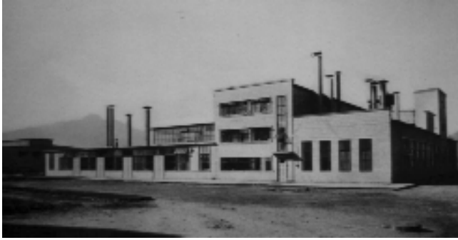
repair house in 1935 (photo by C. Edige)
